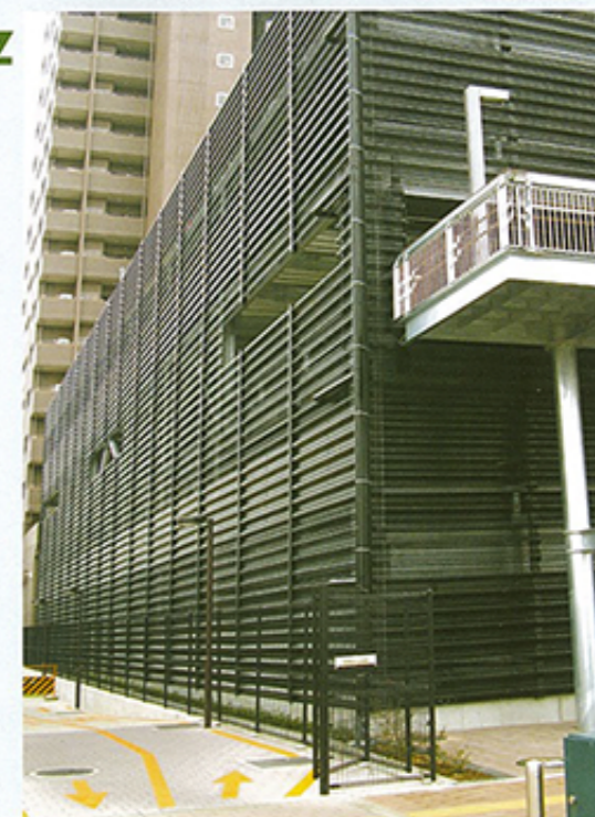
立体駐車場外壁 Exterior wall panels of car parking towers
