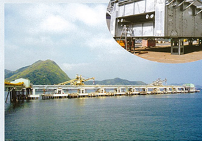
積出し棧橋桁 Shipping pier girders
