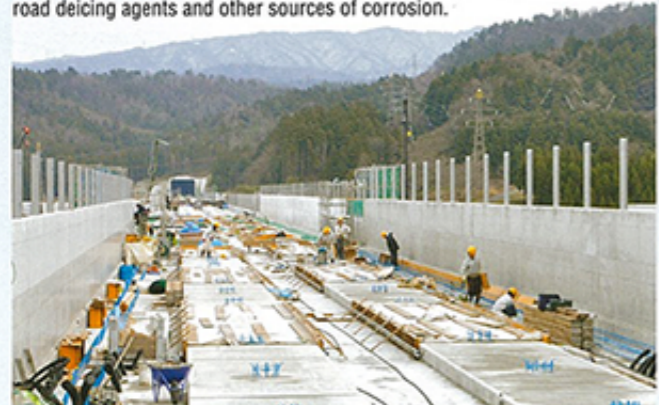
新幹線遮音壁支柱 Shinkansen sound barrier posts
